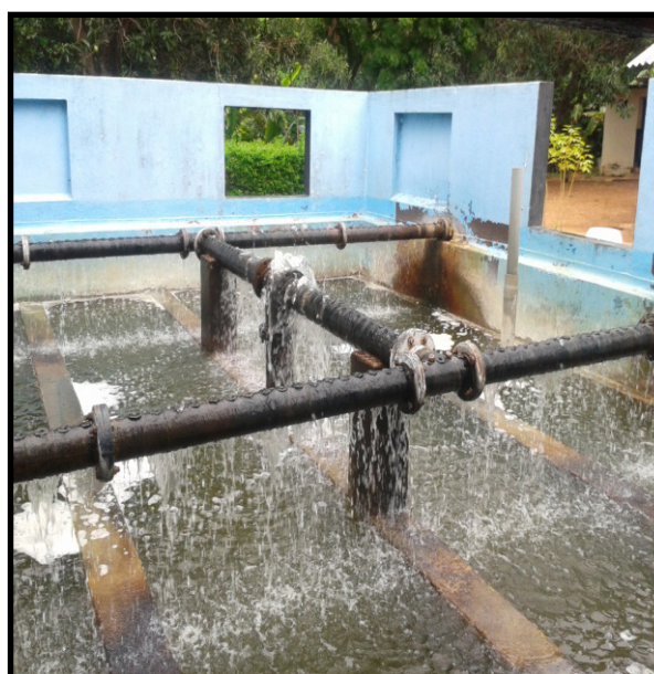
Figure 3: Aeration tank at Andankulam
